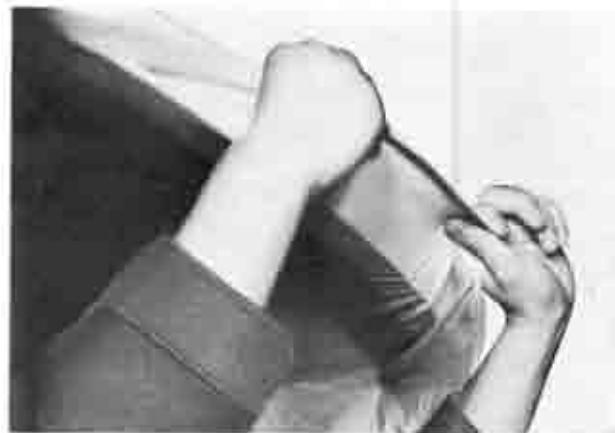
Fig. 14-14 Installing top ceiling
