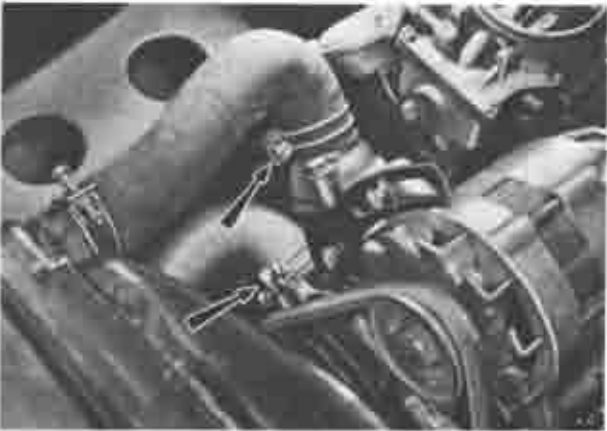
Fig. 1-8 Removing water hoses
