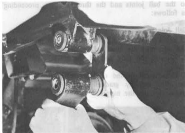
Fig. 13-11 Installing shackle pin
