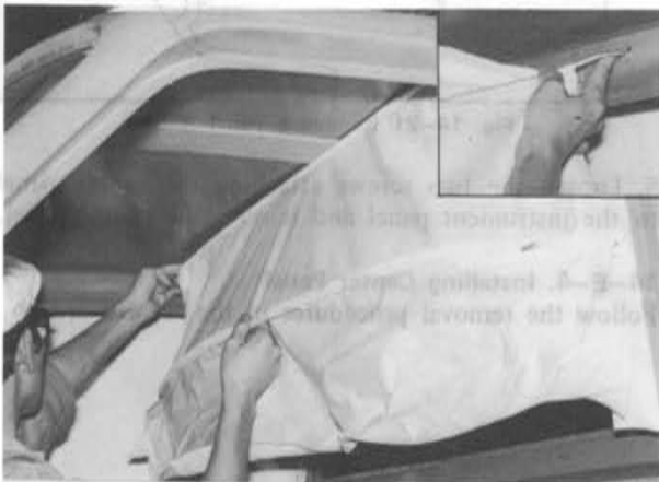
Fig. 14-14 Installing listing wire bracket
