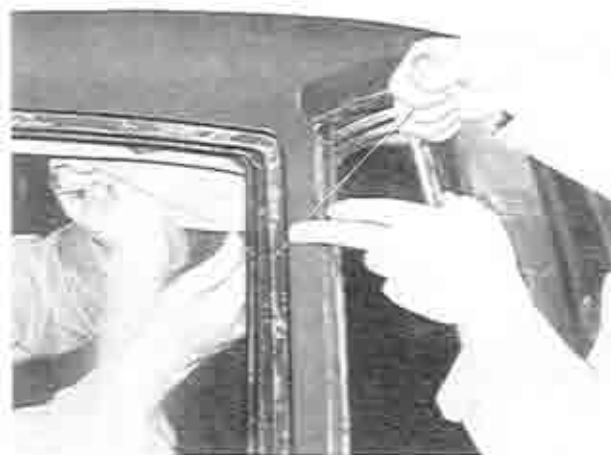
Fig. 14-5 Cutting of sealant
