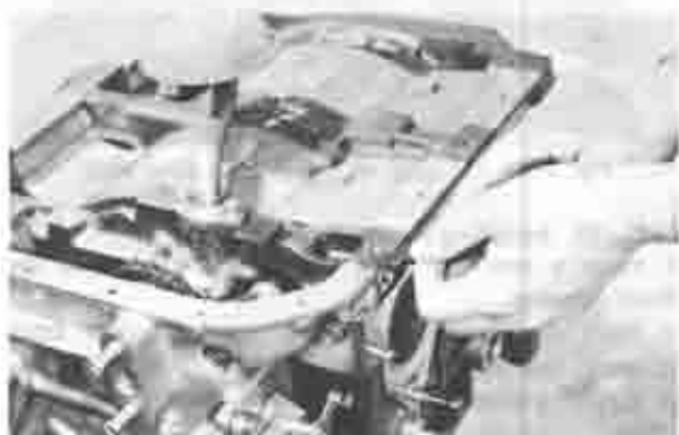
Fig. 1-88 Cutting off excess gasket
