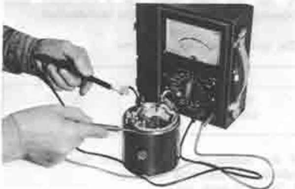
Fig. 5-27 Checking field coil for ground
