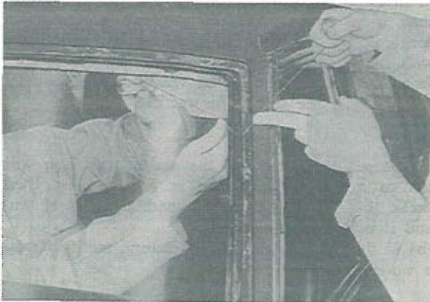
Fig. 14-23 Cutting of sealant
