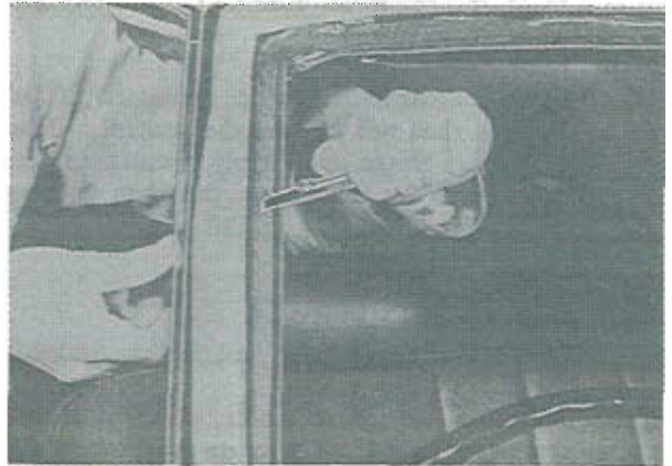
Fig. 14-25 Cutting of sealant
