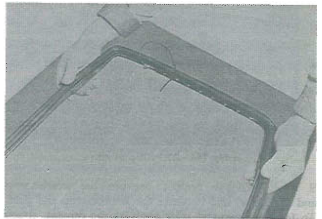
Fig. 14A-18 Installing of weatherstrip
