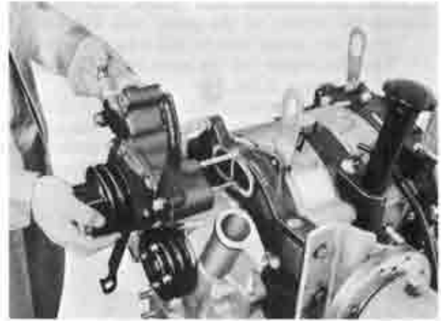
Fig. 1-92 Installing water pump
