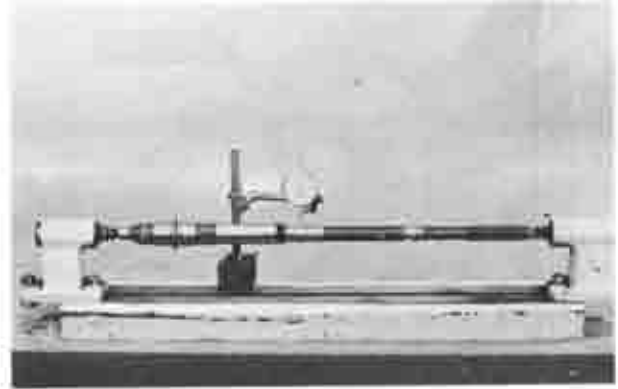
Fig. 7C-33 Checking main shaft run-out
