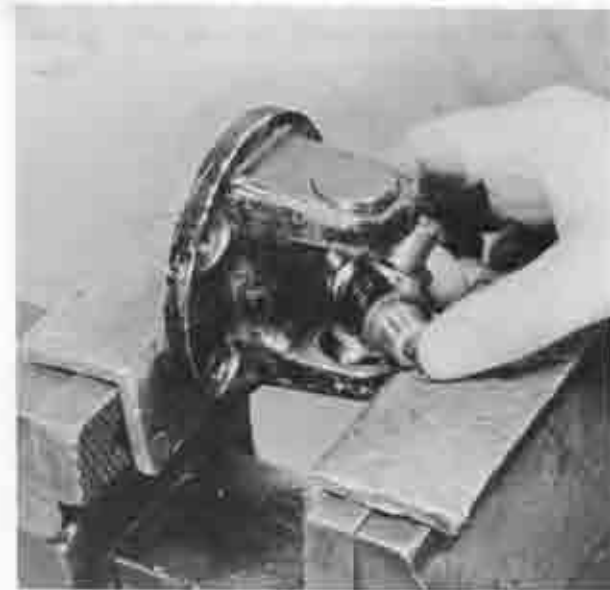
Fig. 8-18 Installing spider
