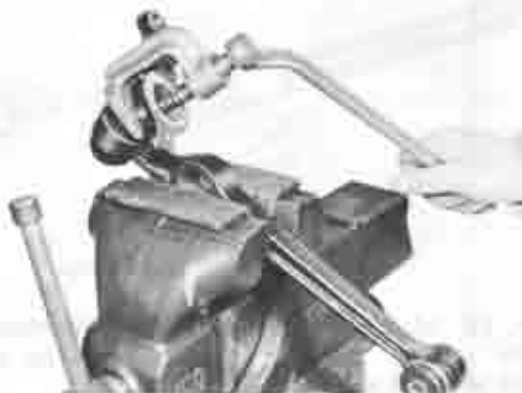
Fig. 13-31 Disconnecting knuckle arm
