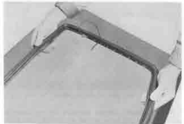
Fig. 14A-19 Installing weatherstrip
