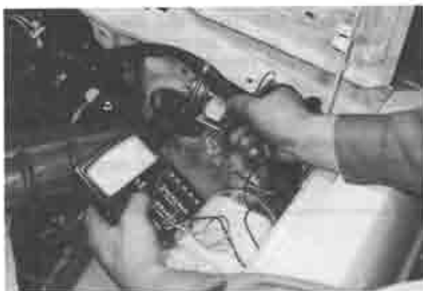
Fig. 1A-28 Checking No.2 vacuum switch
