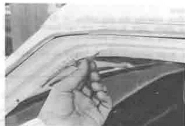
Fig. 14-88 Tearing of ceiling cemented surface
