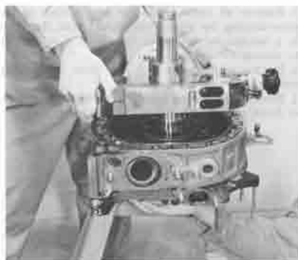
Fig. 1-23 Removing intermediate housing
