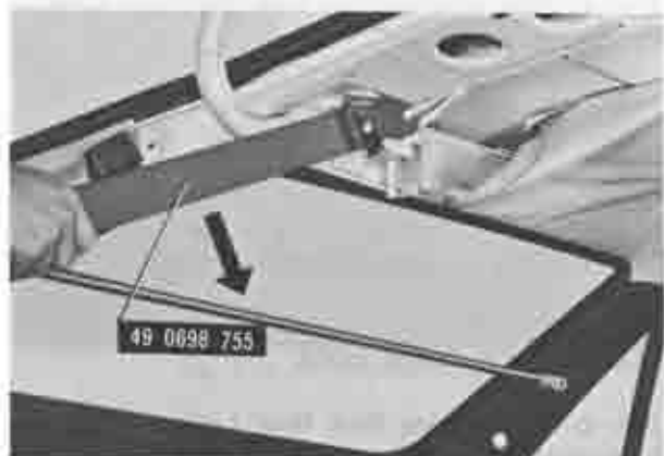
Fig. 14A-12 Installing torsion bar arm
