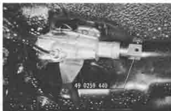
Fig. 7-1 Installing main shaft holder
